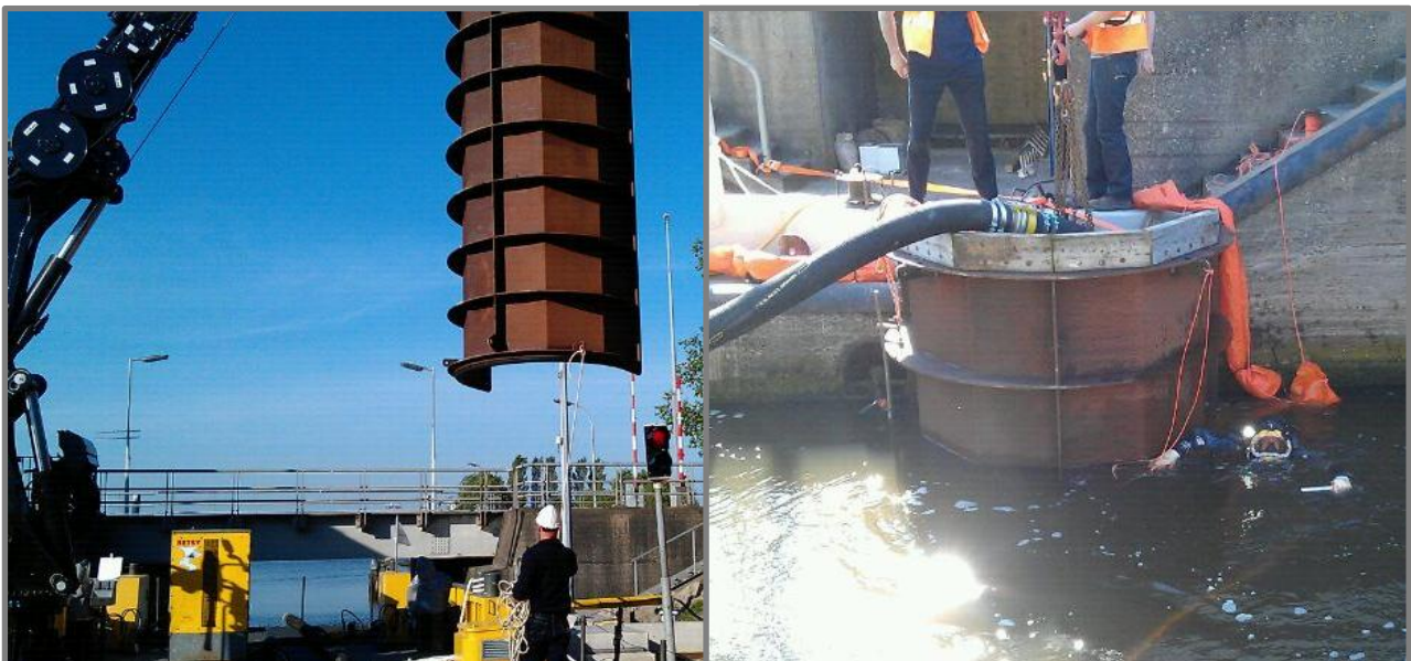
Figure 49: Pictures of pivot-inspection chamber.
