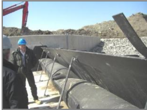
Figure 71: Movable sill. Driving mechanism: Rubber bellow.
