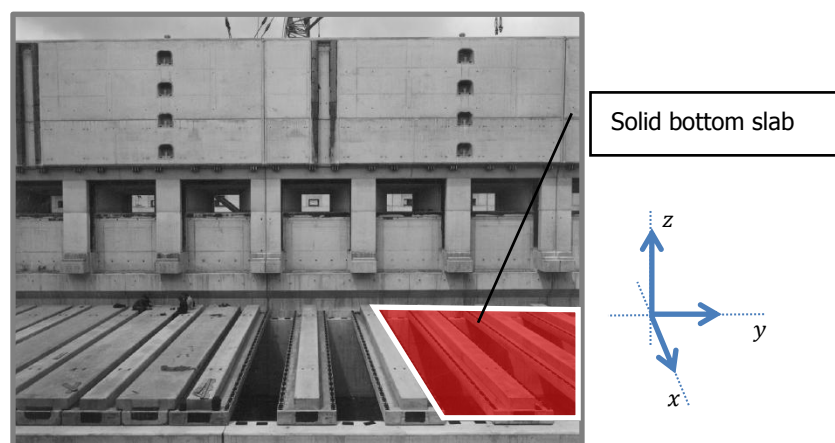
Figure 33: Photograph of bottom slabs in lock chamber. Adapted from (Rijkswaterstaat Bouwdienst, 2000b).
