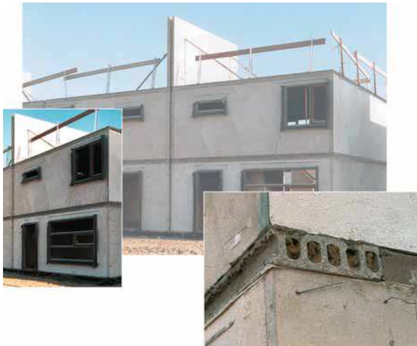
Figure 5-7: Construction single family-dwelling (Source: BFBN)
