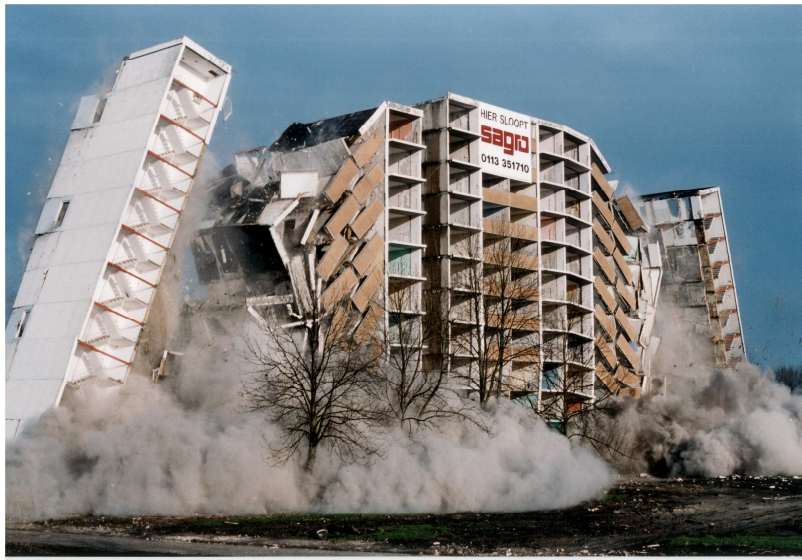
Figure 3-2: Collapse like a house of cards after using explosives to demolish a prefab concrete building in Middelburg (1986)
