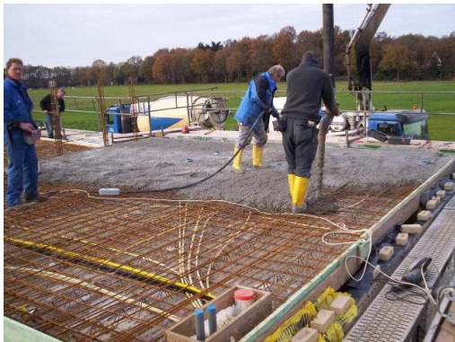
Figure 2-8: In-situ poured concrete system
