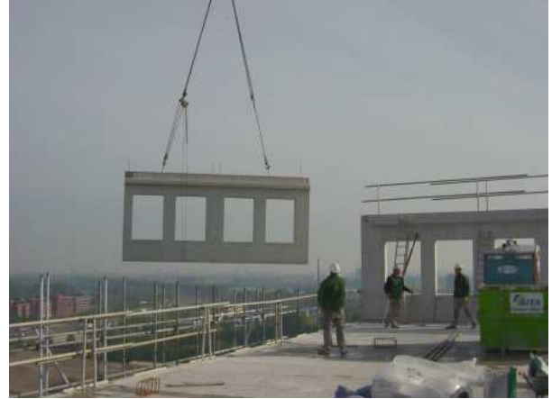
Figure 5-4: Photo 1 constructie PWC (Source: Hurks Beton)
