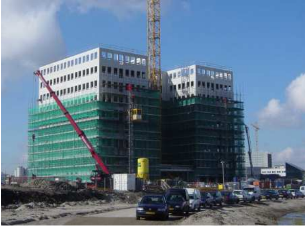
Figure 5-3: Photo 2 constructie PWC (Source: Hurks Beton)
