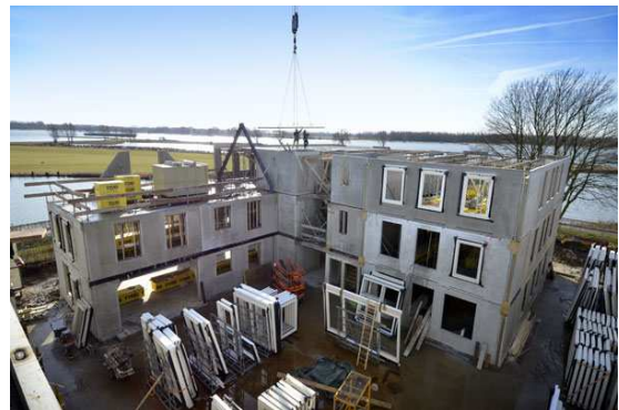
Figure 2-7: Assembly construction system
