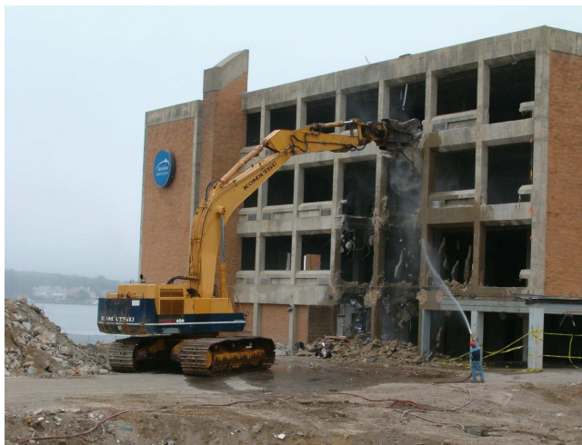
Figure 1-1: Demolition of a building with concrete structure
