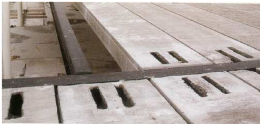
Figure 4-6: Block-outs made at the building site (source: Dycore)
