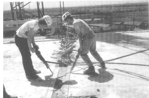
Figure 2-10: Pneumatic hammers project Middelburg
