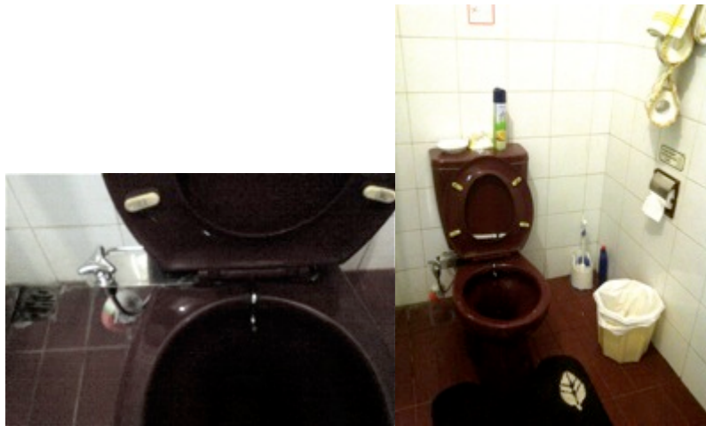
Figure 23 - TOTO toilet modified for 'washers'
