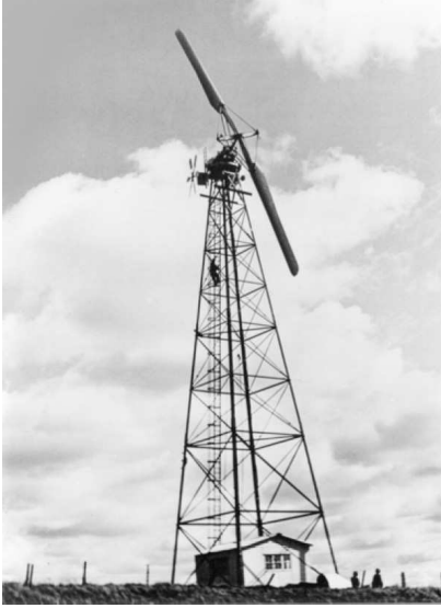
(a) E. L. Smith wind turbine (1941) with a rotor diameter of 17.5 m and rated power of 50 kW.
