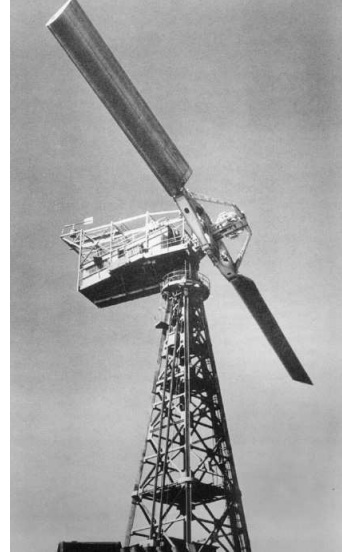
(b) Smith-Putnam wind turbine (1941) with a rotor diameter of 53.3 m and rated power of 1.25 MW.
