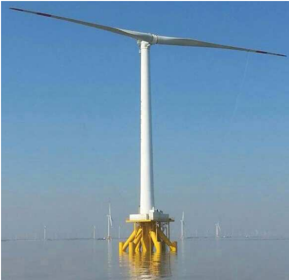
(a) Photograph of the aerodyn 6MW turbine off the coast in China (photograph from (aerodyn engineering GmbH, 2014)).
