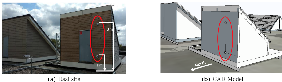
Figure 3.18: Figure (a) Depiction of outdoor experiment setup in Solar beat facility test, Eindhoven. Note that two pyranometers are installed at 1m and 3m from the ground respectively. Figure (b) shows the Sketchup drawing of the site that has been used to retrieve the cartesian coordinates of the shading object and pyranometers for the model inputs.
