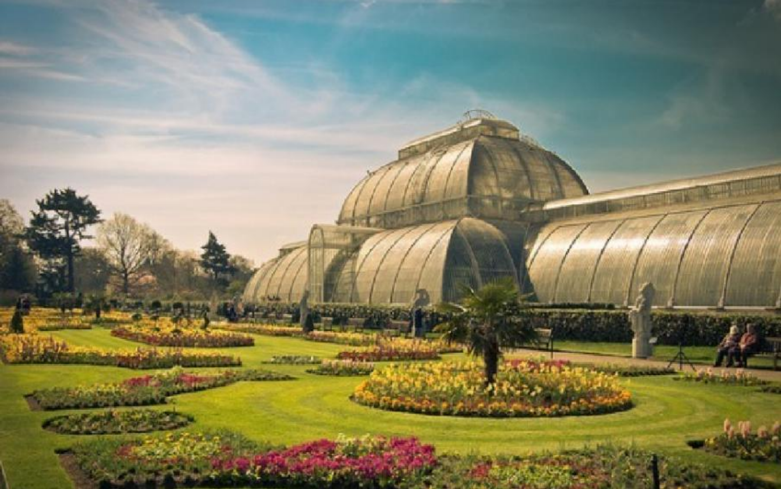
Figure 1.10: Royal Botanic Gardens, Kew, located in United Kingdom. It is a typical green garden architecture, which used curved glass directly connected to steel frames. It expressed the uniqueness of glass that combined both practical and decorative.
