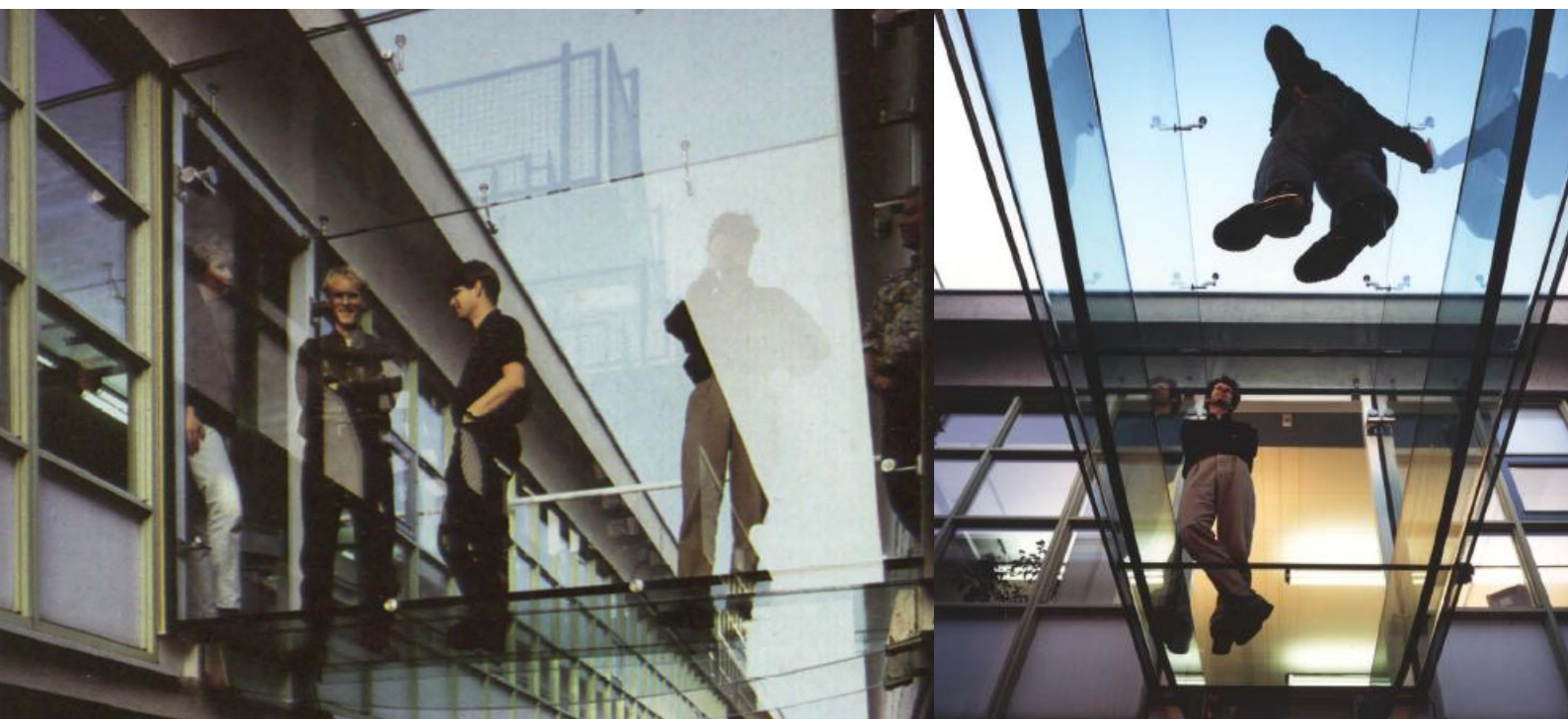
Figure 1.16: the glass bridge in Rotterdam, design by ABT, The Netherlands.
