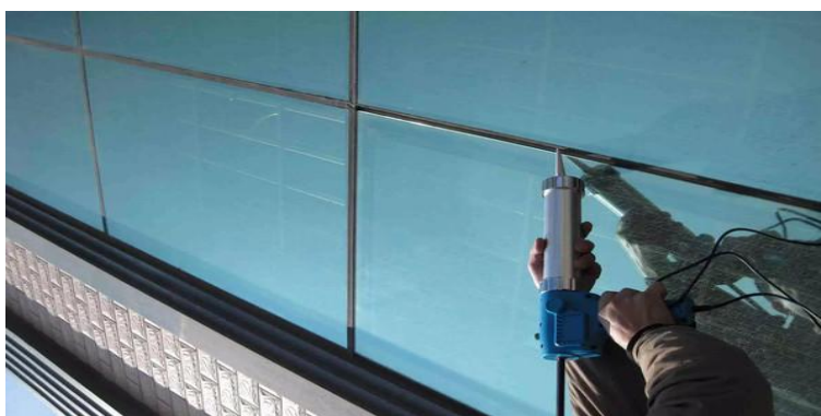
Figure 2.4: Glass adhesives. Glass adhesives are special binders which make strong connections among glass components or between glass member and other substrates, such as metal frame, plastic frame or connectors.
