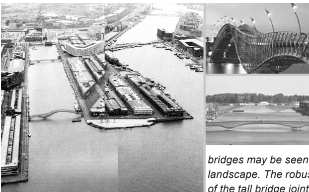
Fig.4-37 The cycle/pedestrian bridges between Borneo and Sporenburg in the Eastern Docklands redevelopment zone of Amsterdam, by West8 Urban Design & Landscape Architecture, won the Footbridge Award for 2002. The bridges were nominated in the Aesthetics (medium span) category on account of their distinctive visual design and their engineering detailing. The jury had several reasons for awarding the prize to these bridges: "The visual unity of the two pedestrian bridges may be seen as an artistic element in the Amsterdam docks landscape. The robust, taut quality of the low bridge and the eccentricity of the tall bridge jointly have an imposing effect on the surroundings.
