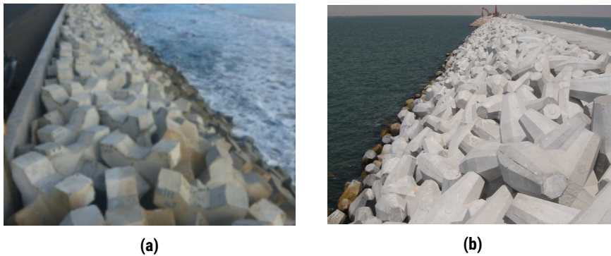
Figure 2.2: a) Xblocs used as armour layer, ( www.xbloc.com ) b) Core locs used as armour layer, ( www.concretelayer.com )
