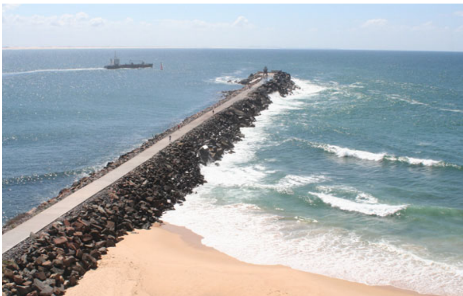
Figure 1.1: Nobby's breakwater, Newcastle (R. Foong (2013))
