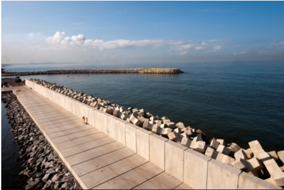
Figure 1.2: Crown wall on top of a breakwater at Dikkowita Port ( www.xbloc.com )
