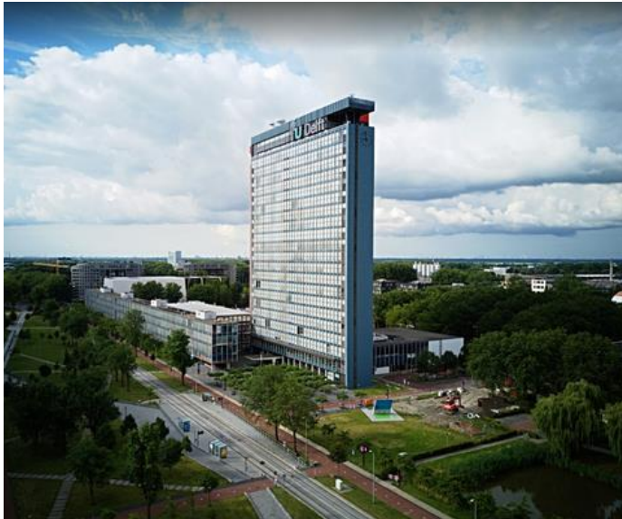
Figure 22: Photo of EEMC in Delft (aerial view) [41]
