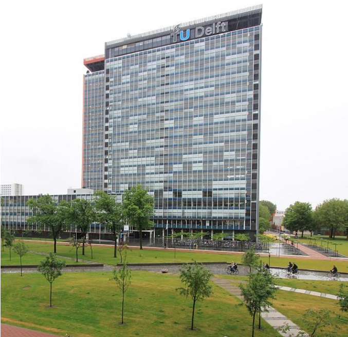
Figure 21: Photo of EEMC in Delft (from ground level) [52]
