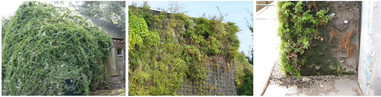
Figure 3. Examples of possible damages due to the lack of maintenance and to design mistakes.
