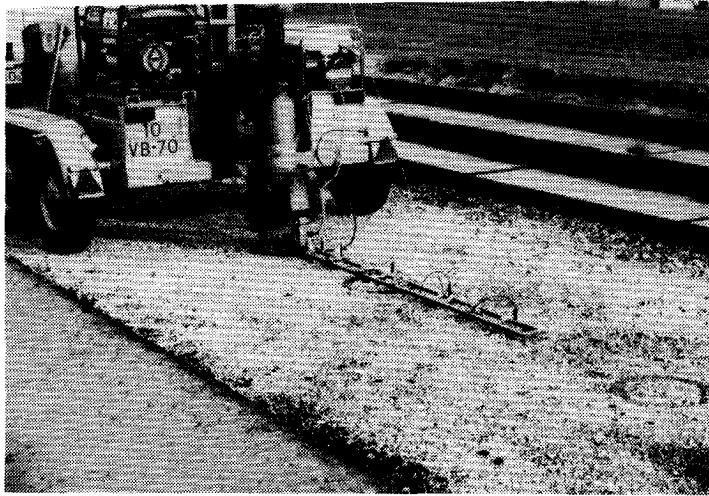
Figure 8.14: Detail of geophones on granular base.
