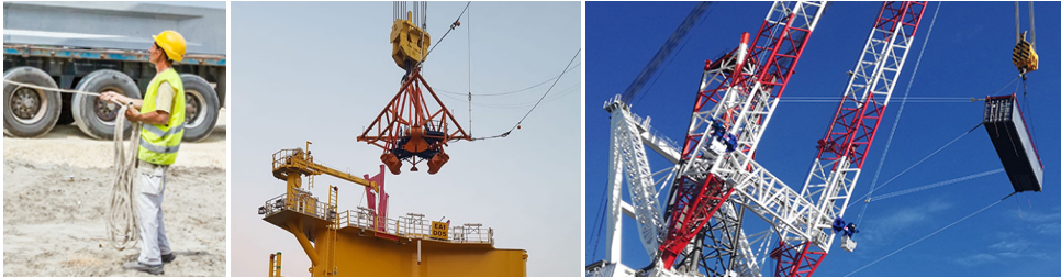
Figure 1.12: Usage of taglines during lifting; manual control [l], attached to lifting gear [m], automatically controlled system [r]
