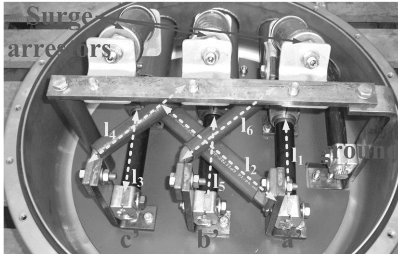
Figure 5.13 Inside view of the CB-box.
