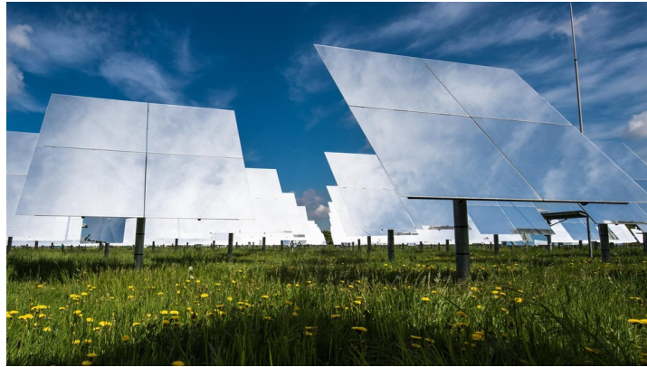
Figure 4.4: Example of a real heliostat at the Jülich CSP plant. Each heliostat consists of four flat rectangular facets that are slightly canted toward one another to concentrate sunlight onto the receiver. [23]
