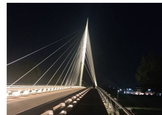
Img 3. Bridge as an example of a liminal space
