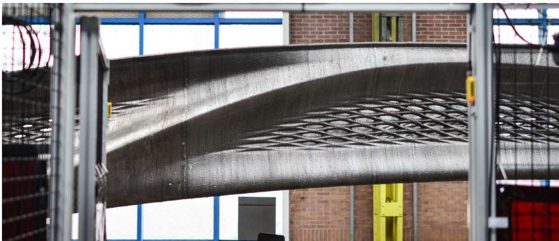
Figure 11 Close up of printing layers and texture bridge (De Groot, 2018)
