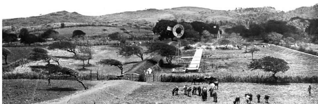
FIG. 15 Windwaterputten (wind-water-well) with series of water reservoirs in the valley of Plantation Savonet around 1900. Between the cattle and the water system a rooi is situated. Large earthen dams are built around the premises as water catchment system. In the hof divi divi trees are planted. Photographer: Soubllette et Fils. Source: RCE.
