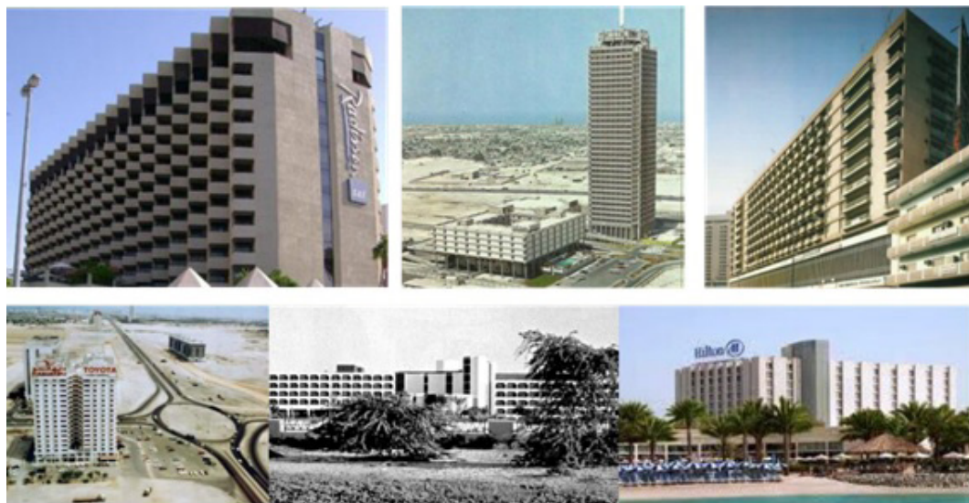
FIG. 9 Examples of modern buildings in Dubai from the period (1960s-1970s).
