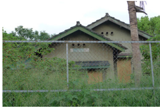
FIG. 16 Shuijiaoshe Village in Tainan City, one of 13 MD village cultural parks established by the Ministry of National Defense, awaits restoration. Source: Photographed by Szu-Ling Lin in 2015
