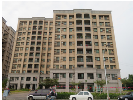
FIG. 13 A reconstructed MD village in Pingtung City. Source: Photographed by Szu-Ling Lin in 2018
