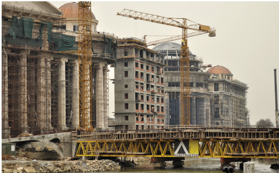
FIG. 2 Skopje city centre, project "Skopje 2014" in construction. Source: (authors archive)
