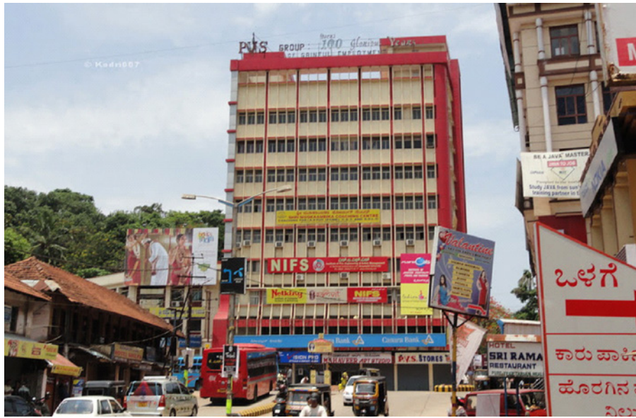
FIG. 9 The first high rise building of Mangaluru built in Kodialbail in 1976.. Source: [Image of PVS Building in Mangaluru](2018) Retrieved from https://www.skyscrapercity.com/showthread.php?p=78718120
