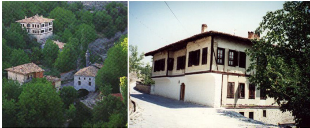
FIG. 9 Environment of Haci Huseyinler house. Source: (Harputlugil and Cetinturk, 2005)
