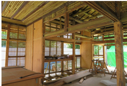
FIG. 24 Environmental sustainability aspect: Building restoration. Source: Photographed by Szu-Ling Lin in 2018
