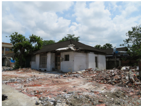
FIG. 32 Authenticity issue: Many additional structures built by the residents of the MD villages were removed after conservation. Source: Photographed by Szu-Ling Lin in 2017
