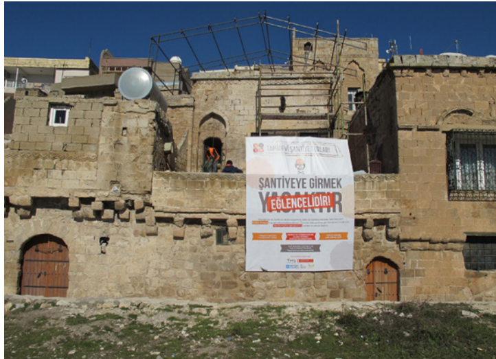
FIG. 1 Tamirevi's southern façade. Source: KMKD Tamirevi Archive
