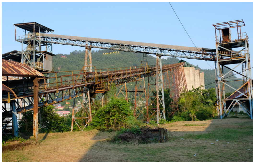
FIG. 5 Former coal conveyor belt. Source: author, 2019.
