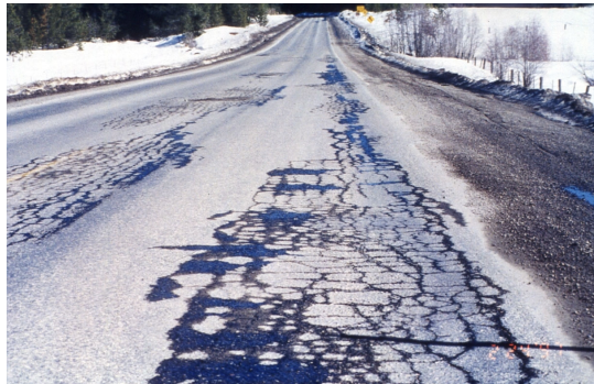
(a) Pavement cracking due to freeze-thaw cycles 1
