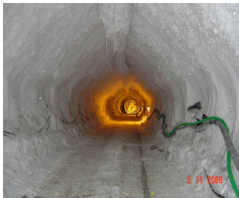
(a) View of frozen ground in a tunnel in Sweden
