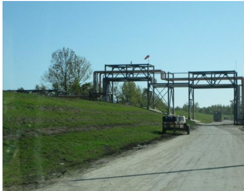
Figure 3-9 Pipelines crossing the Mississippi Levee [Report: M903703_site_investigation_stolt_nielsen]
