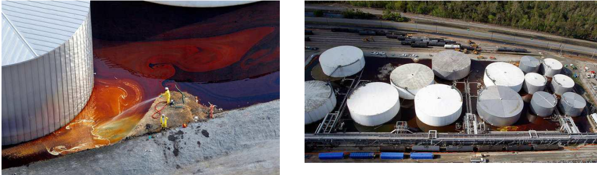
Figure 3-10 Spill of chemicals on the terminal [18]
