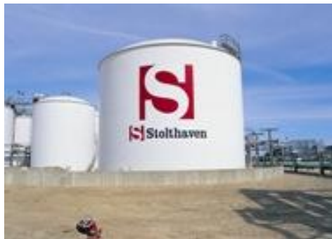
Figure 2-3 Example of a steel storage tank [ http://www.stolt-nielsen.com/Stolthaven-Terminals.aspx ]
