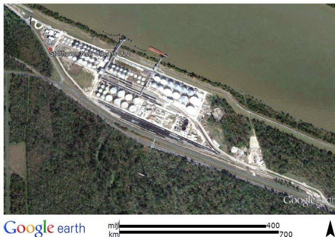
Figure 3-8 Storage tanks on the existing terminal site
