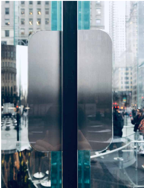
FIG. 4.50 Laminated fitting in fin and face glass with offset stainless steel plate connection
