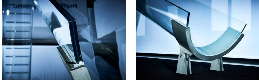
FIG. APP.A.13 Base detail with stainless steel shoe fixed to glass surface with structural silicone
