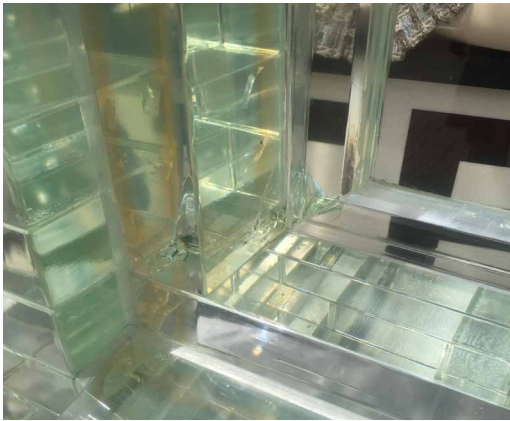
FIG. 3.68 Crystal Houses, Amsterdam, window frame and sill.
