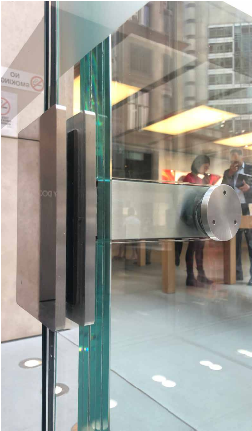
FIG. 3.45 Clamped fitting George street (comparable to CB1)
