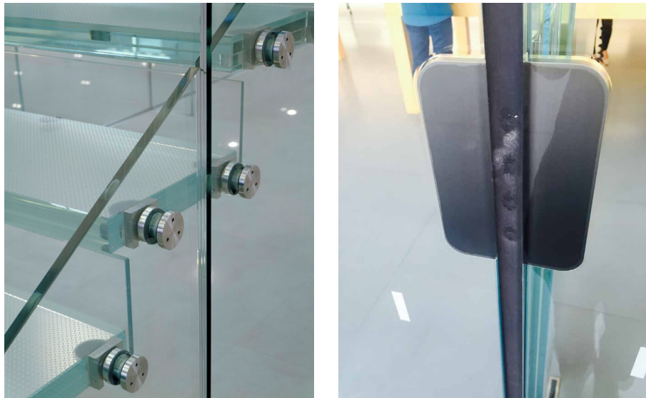
FIG. APP.A.8 Typically glass structures consist of many layers of glass, connected with opaque fittings that transfer the load.
