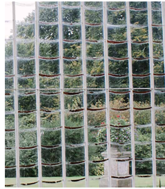
FIG. 3.11 Close-up of 2-side supported overlapping shingles
