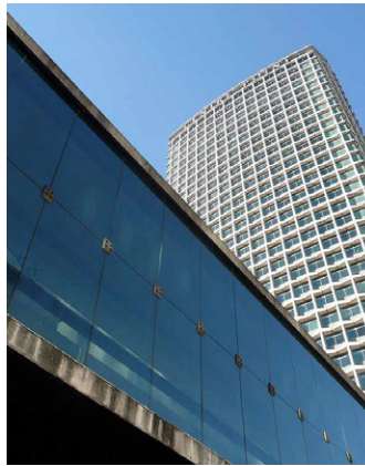
FIG. 4.31 Centre Point Link bridge clamp fittings
