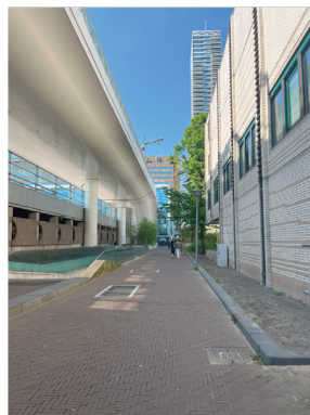
6: Going straight, walking between the railway and National Archives building.
