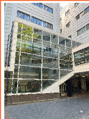
13: View of entrance from the other side, very hidden.
