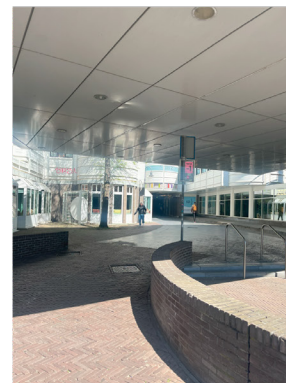
9: Passing under the tram viaduct.
