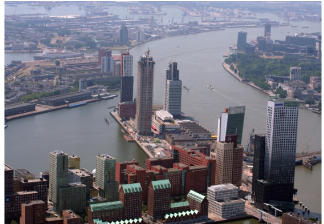
Fig. 66 Picture of the Kop van Zuid at the river Maas (RTV Rijnmond, n.d.)
