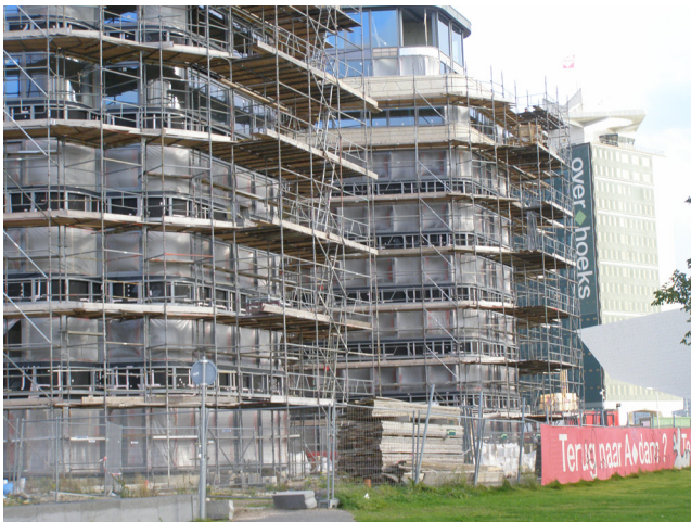
Fig. 52 Apartment buildings Overhoeks (author, 2011)
