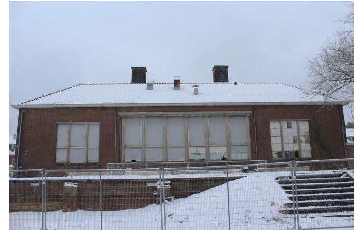
West façade, “original back”
