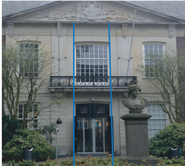
Fig 5.21 Facade Maternity Clinic Vertical orientation because of white window frames own illustration
