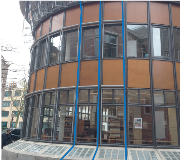
Fig 5.20 Facade Administration Building Vertical orientation because of the shape of the panels and glass. own illustration
