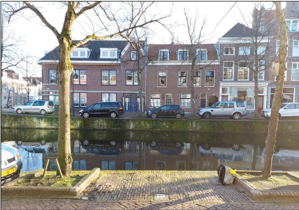
Picture 46: shows the location of the quay walls of site 8 (own picture)
