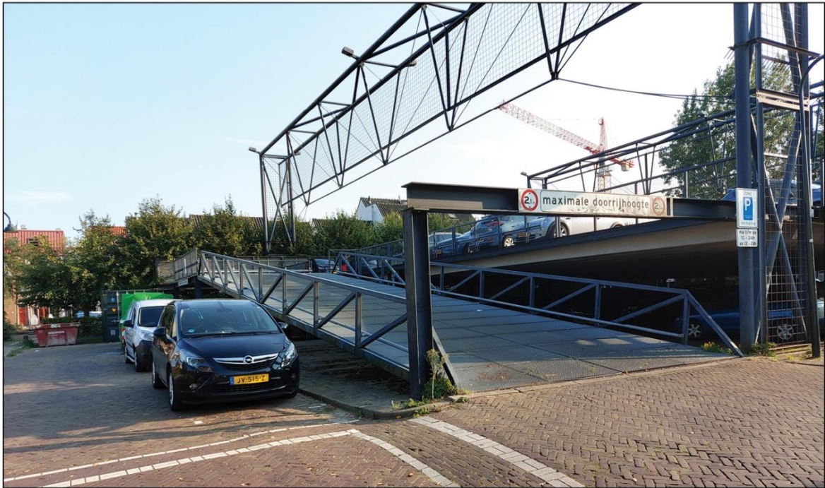
Picture 1: Location of site 1, underneath the steel slope bridge (own picture)
