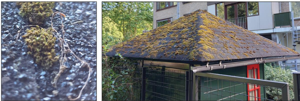
Picture 31: left side is a close-up view of the cushion moss and the right side shows the east and north-facing direction of the roof slope (own picture)
