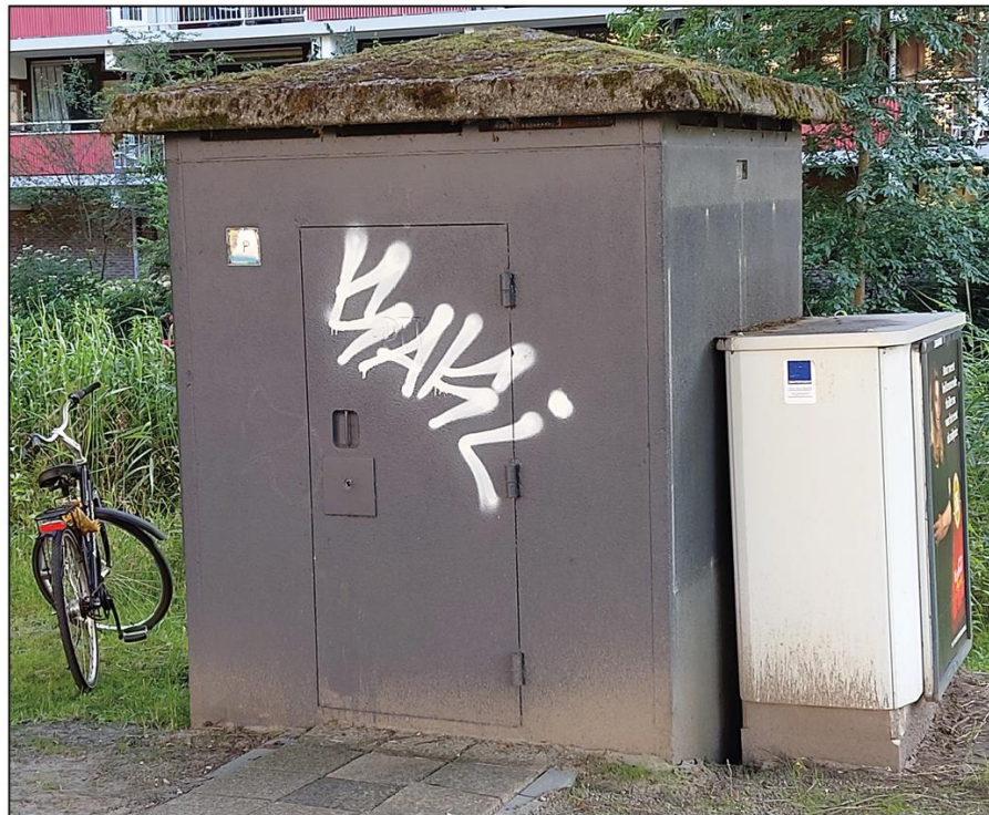
Picture 6: Location of site 2, the cementitious roof of the powerhouse (own picture)
