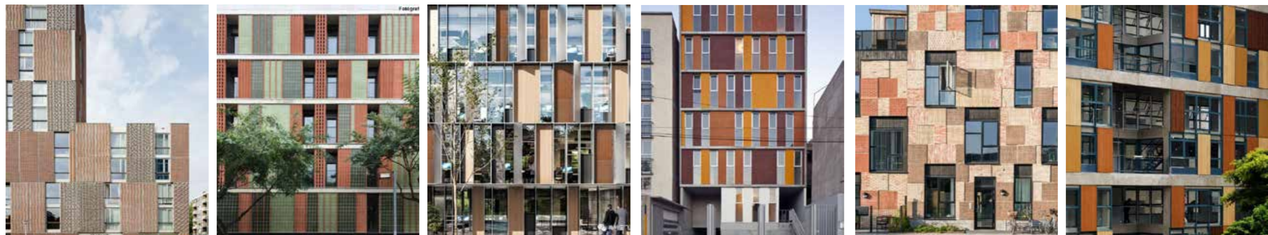
In designing the facade, I explored different rhythms that could be repeated throughout the building. The ground floor features the widest rhythm.
