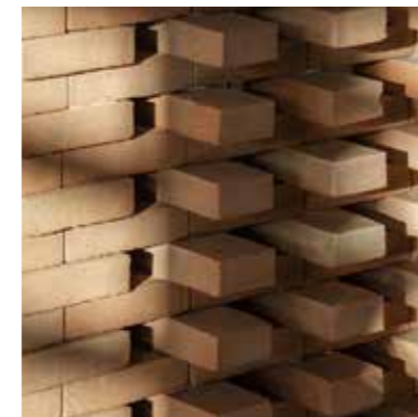
Bricks made from demolition waste
