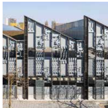
Steel contour plates residual material from the automotive industry
