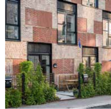
Brick Recourse rows, Lendager
