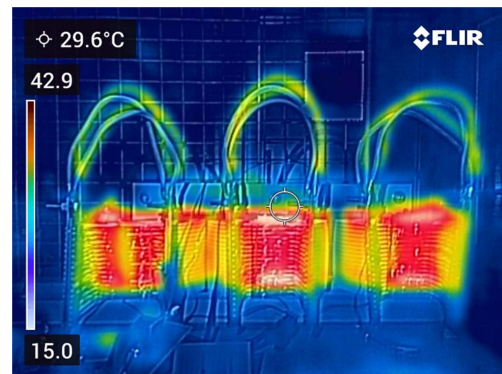
FIGURE 17. Infrared thermography image of the fabricated three-phase MFT during operation.
