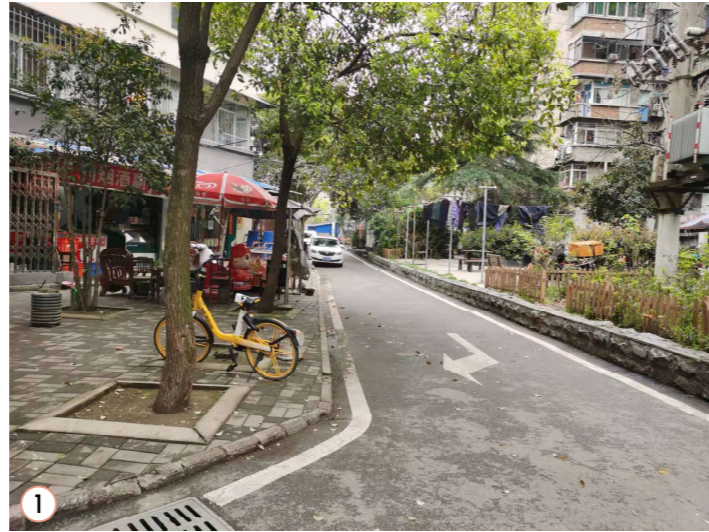
2 Deteriorated street infrastructure
