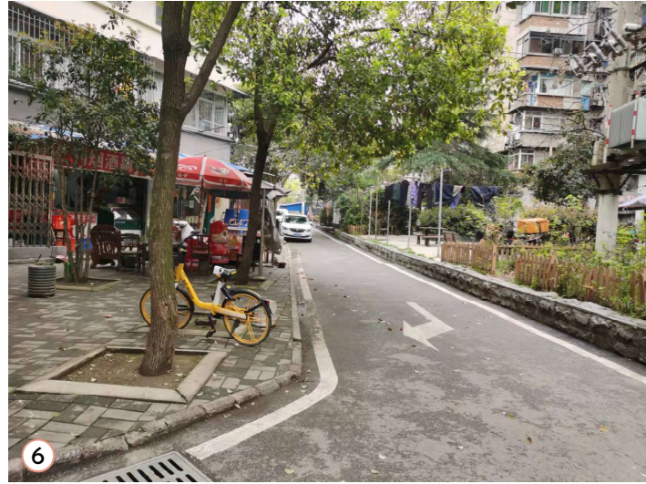
6 Deteriorated street infrastructure
