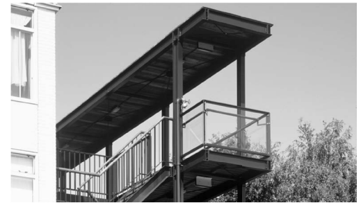
Fig.25. External view of the new gallery.
