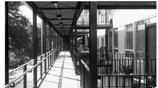
Fig.26. The inside of the new gallery with bridges to the front doors.
