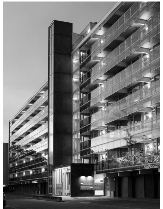
Fig.24. The new facade and elevator.
