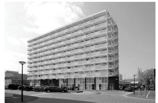
Fig.21. Frissestein smaller scale building.
