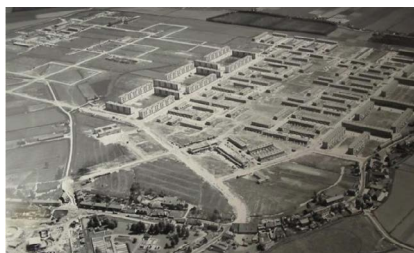
Fig.47. New construction of Hordijkerveld next to the old dike houses.
