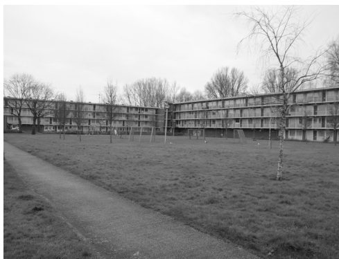
Fig.53. The large open courtyard in-between the gallery flats along the Huniadijk. Also chosen location for the design strategy
