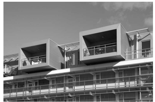
Fig.23. The penthouses on top of the old roof.
