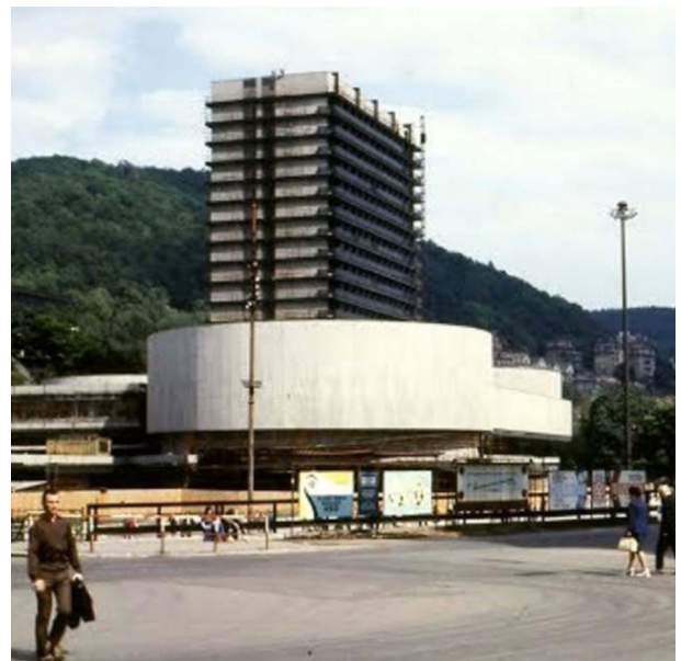
Figure 36: Spa Hotel Thermal in 1977, Karlovy Vary (Spa Hotel Thermal, n.d.)
