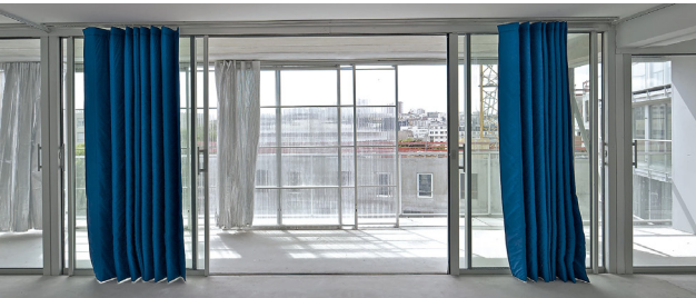
Social housing renovation Paris by Lacaton & Vassal (Ruault, n.d.)
