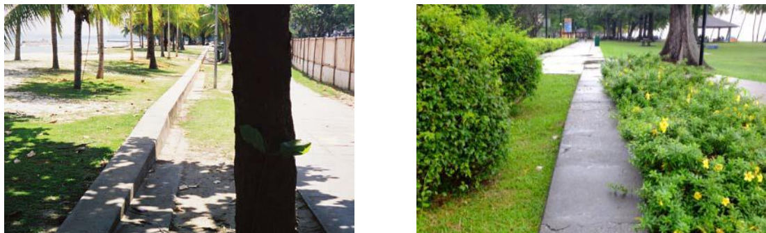
Figure 3.3 Crest of the old seawall still visible along East Coast Park. Left: photo taken by Teh Tiong Sa, 2001. On the image the crest of the seawall is visible, reaching above the ground level. In fact, this ground level had lowered as a result of land subsidence, for which on both sides of the seawall the ground level is lower than the crest of the seawall. Right: Photo taken by author, December 2012
