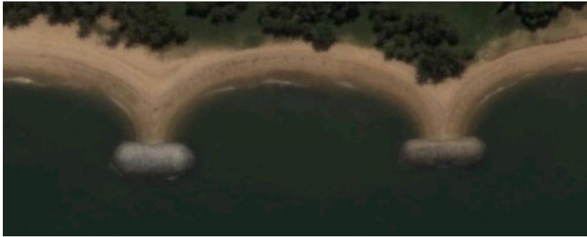
Figure 6.7 Example of a pocket beach along East Coast Park.
