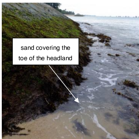
Figure 6.24 Straight beach west of headland 6. The dashed red circle indicates the location and direction of the photos below. The lower left photo shows sand surpassing the headland, and the lower right photo shows the retreat of the water line seaward of the headland.
