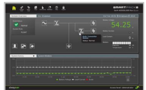
STATUS OF DC/DC CONVERTERS IN SMARTPACK2 WEB
