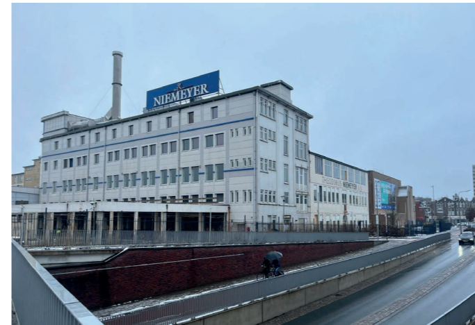
F28. AI factory in the old Niemeier building
