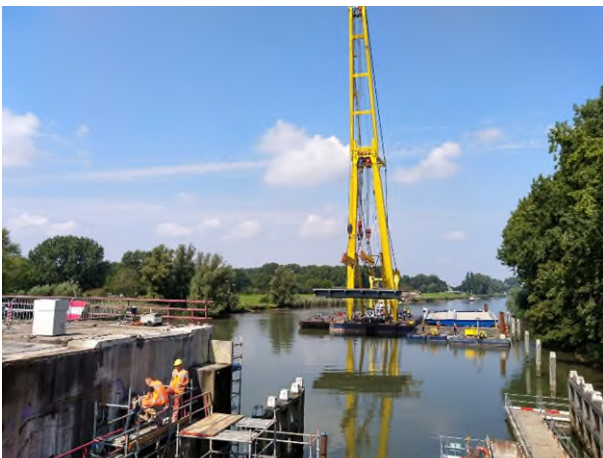
Figure 7. The lifting of the bridge deck.
