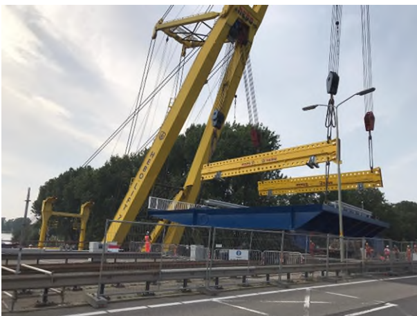
Figure 8. The lifting of the bridge deck.
