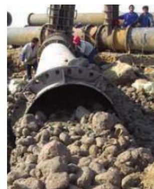
Figure 70: The formation of clay balls by pipeline transport (source: Van 't Hoff & Van der Kolff, 2012)
