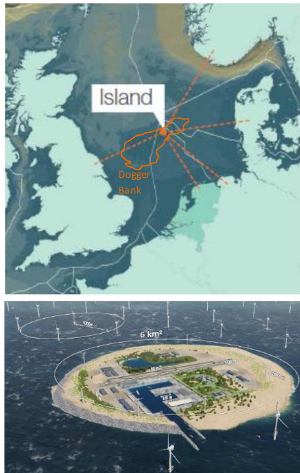
Figure 8: The hypothetical location on the Dogger Bank of the energy hub with its interconnector cables indicated with the dashed lines (top) and an impression of the envisioned island by TenneT (bottom). The figure was modified from Van der Hage (2017) and Börger et al. (2014)
