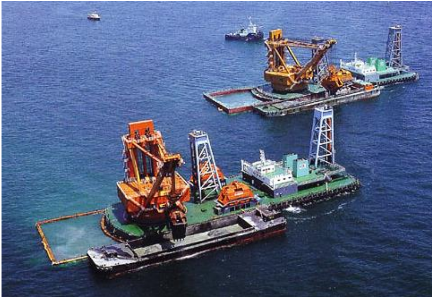
Figure 78: Silt screens directly attached to the grab dredgers. Note the difference in turbidity in- and outside the silts screens (source: https://nippon.zaidan.info/seikabutsu/2000/00736/images/174-1.jpg )
