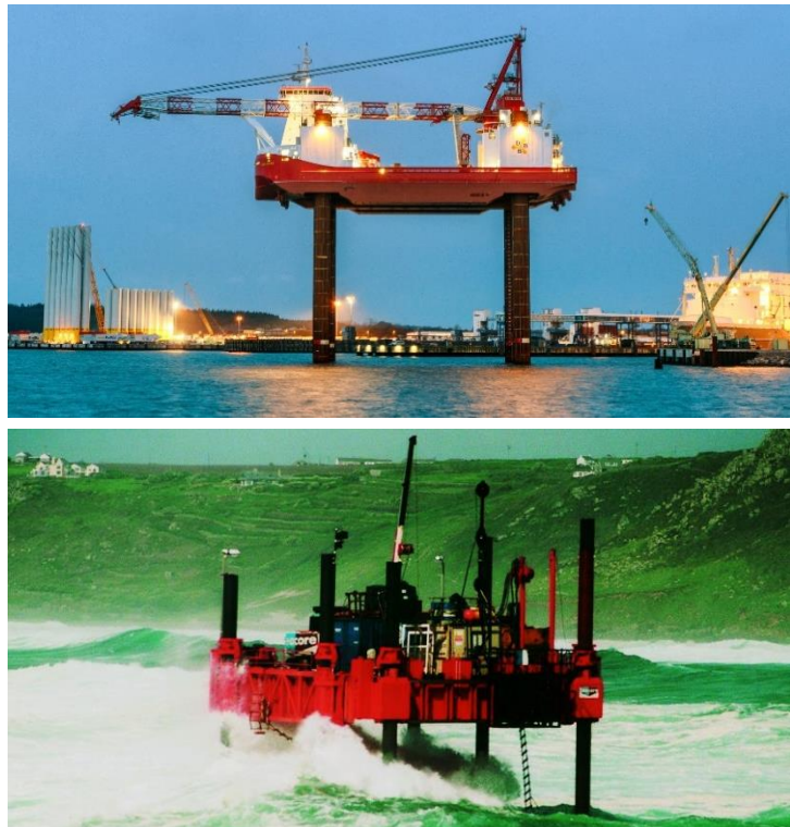
Figure 73: An offshore wind turbine installation vessel performing its jack-up tests (top) and a working platform (bottom) (source: http://www.ziton.eu/wp-content/uploads/WIND-SERVER-jacked-03-low-res.jpg ; http://www.thinkdefence.co.uk/ship-to-shore-logistics/increment-2-pier/ )
