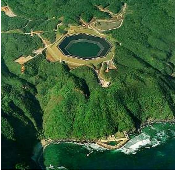
Figure 19: The Okinawa Yanbaru seawater PHS plant in Japan (source: Fujihara et al., 1998)
