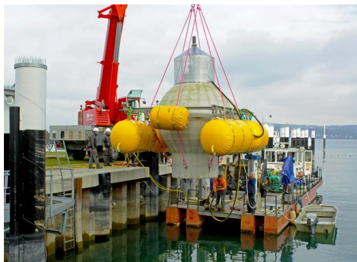
Figure 125: The 1:10 pilot being installed (source: https://www.energiesystemtechnik.iwes.fraunhofer.de/en/projekte/se-arch/laufende/stensea.html )
