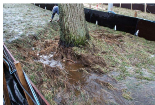
Figure 4-19: Damage NWO tree landward slope
