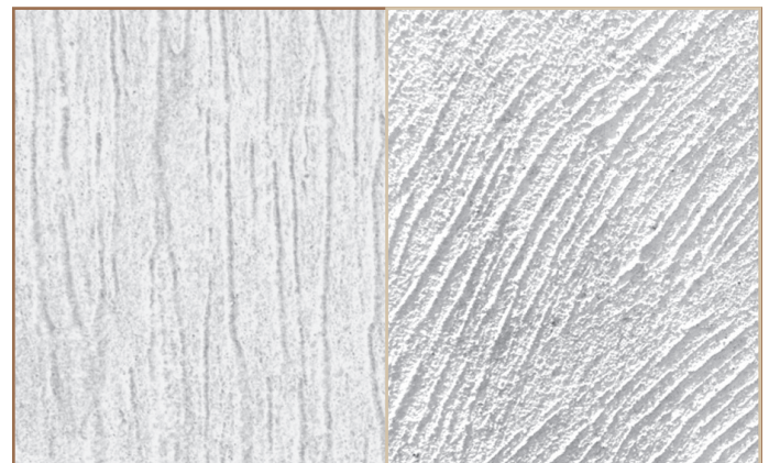
Image 11. Textured wall surfaces, guiding movement throughout the building. (Gallery of School for Blind and Visually Impaired Children / SEALAB - 14, n.d.).
