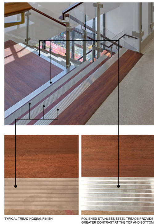
Image 6. Staircase design for the Lighthouse for the Blind and Visually Impaired by Chris Downey and Mark Cavagnero (Image retrieved from Mark Cavagnero Associates Architects).
