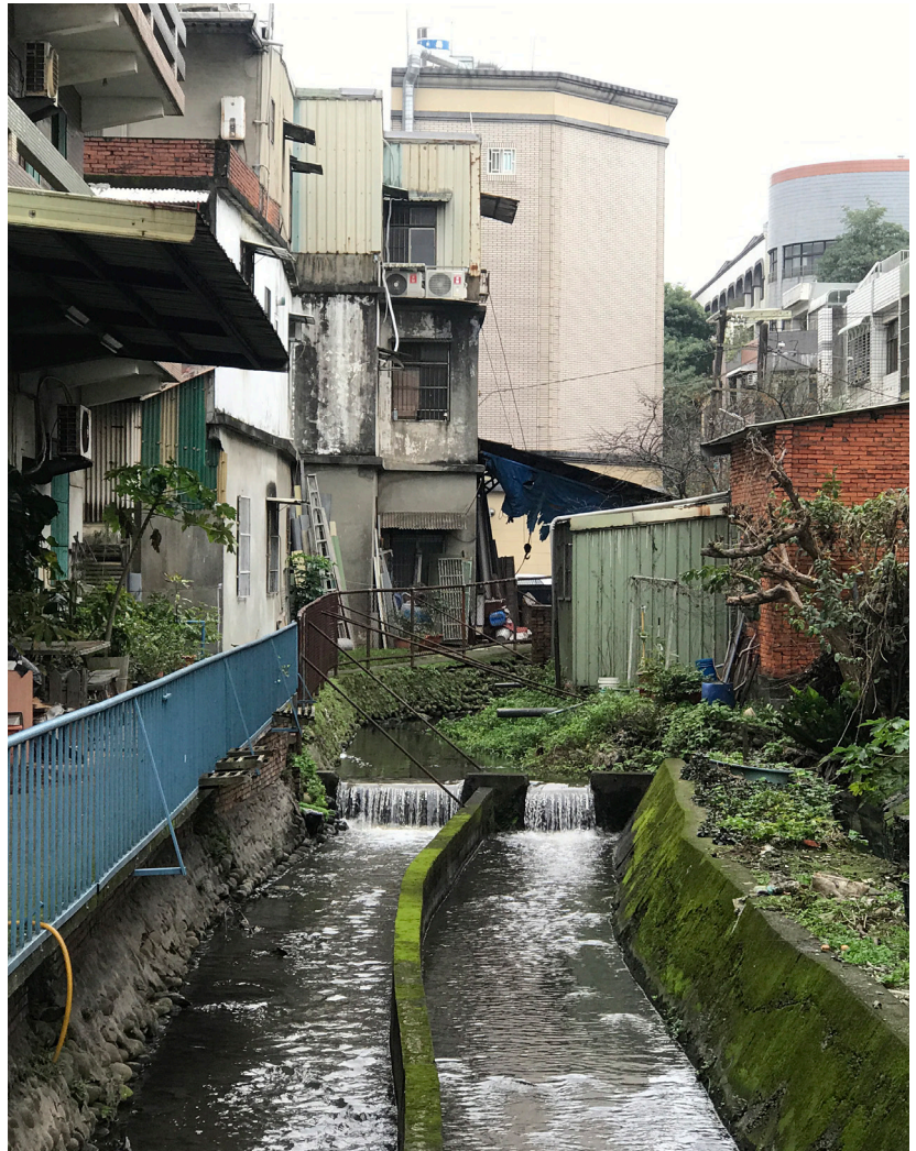
Figure 01-2 Irrigation works in the community Source: Taken by author
