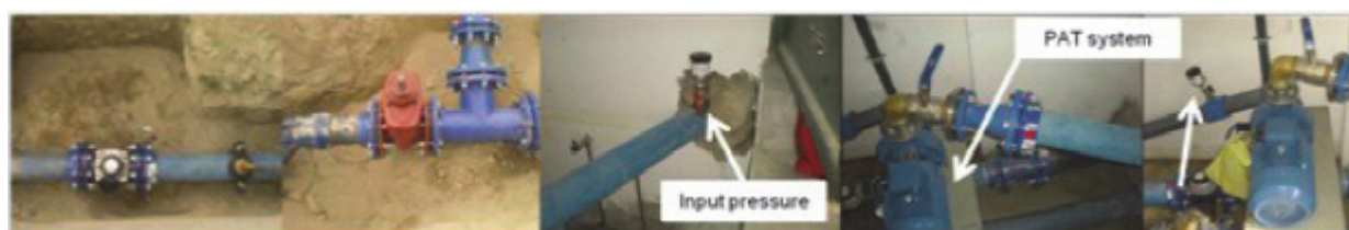
Figure 7-8: System tests in pipes
