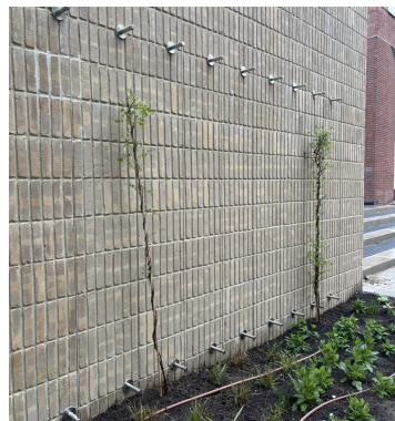
Figure 2.3: Just planted indirect green facade with continuous guides at Naritaweg, Amsterdam (own work)
