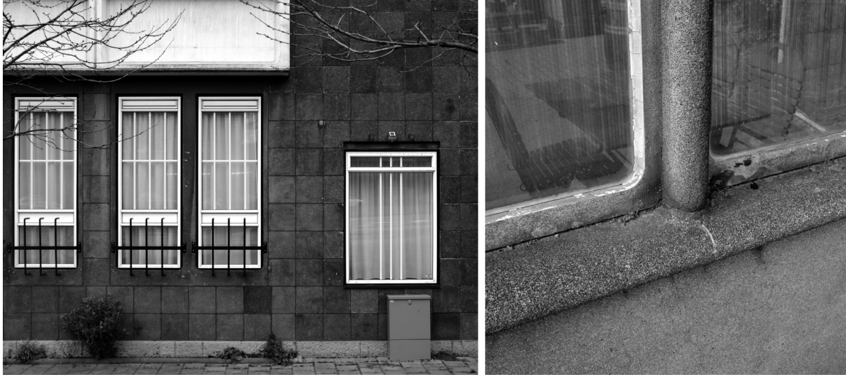
Fig. 2. Left: B. van Veen, Bank and apartment building, Rotterdam, 1939–1940, basalt-Shockcrete. Right: S. van Ravensteyn, Blijdorp Zoo, Rotterdam 1939–1941, brick-Shockcrete. © Wido Quist, 2020, 2019.
