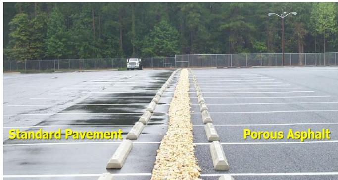
Figure 1.1: Water draining ability of porous asphalt [6].
