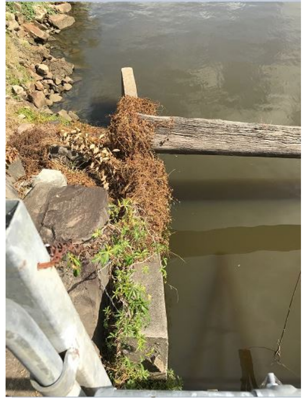
Figure C.2: Current state of the outlet wall of the Floodgate. It is clearly visible that the outlet wall is tilted.
