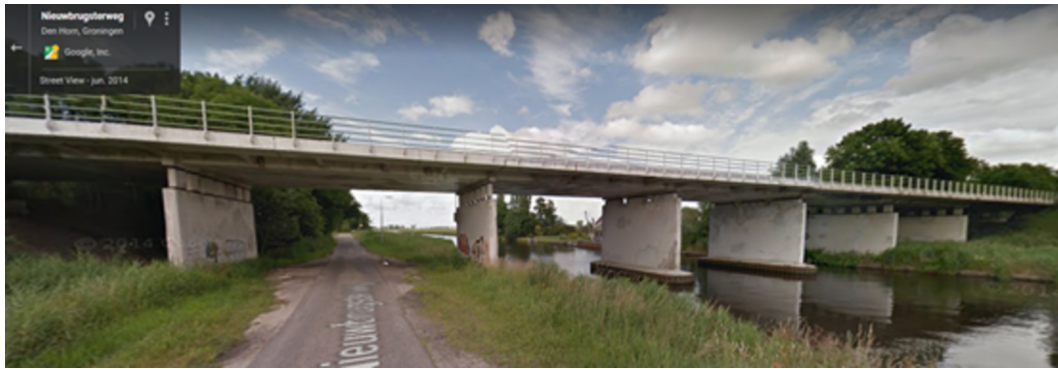
Fig. 5. Google Maps view of Nieuwklap Bridge.
