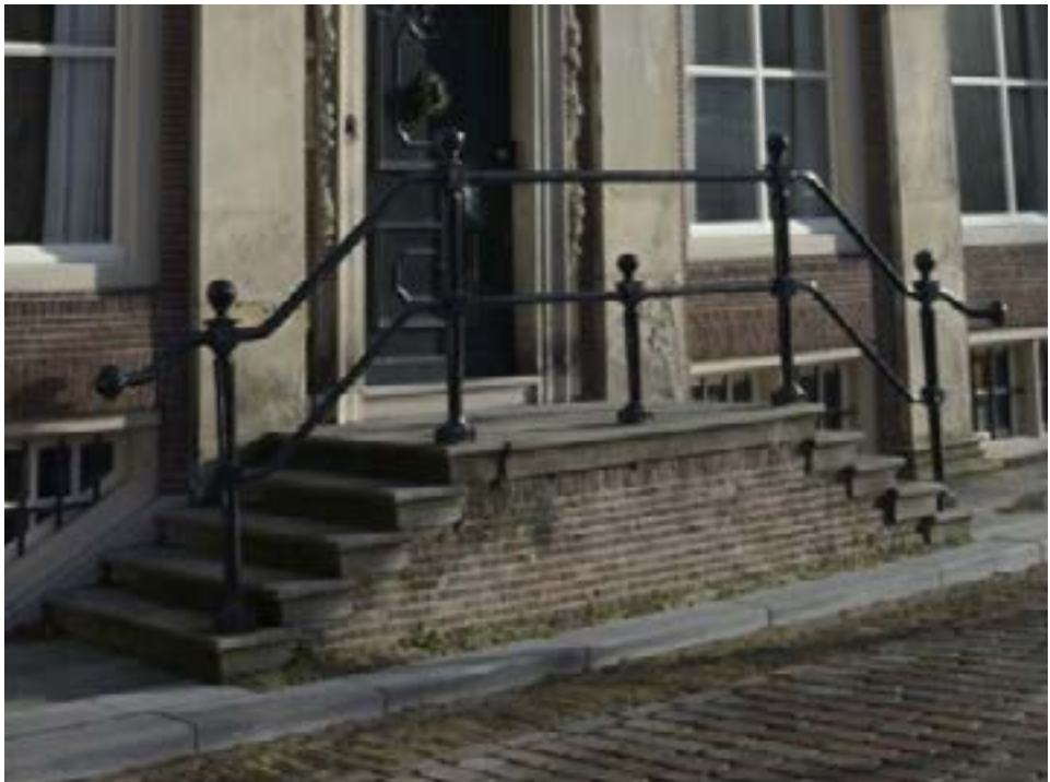
figure 12: Houses at the Korte Engelenburgkade are built to flood only at the basements (Reizen langs rivieren, n.d.)
