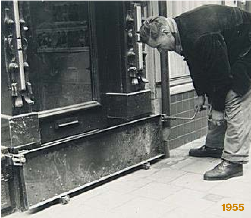
figure 19: Flood-resilient panels being tested in Dordrecht in 1955 and 2021. (Left: Regionaal Archief Dordrecht, 1955. Right: D. Koorevaar, 2021)
