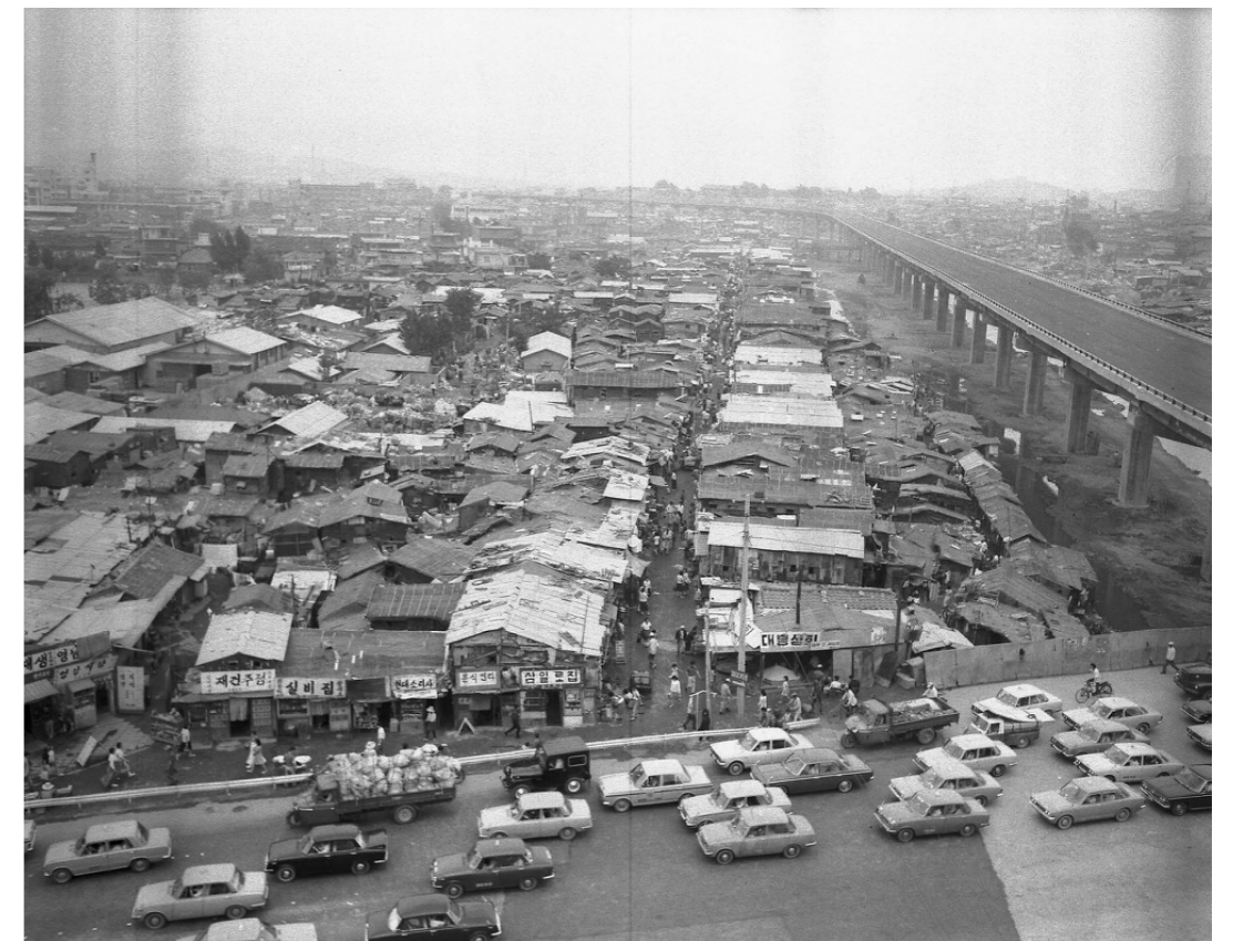
Figure 1.10 Informal structures along Cheonggyecheon (1972). Photograph, archive no. 24620894. Retrieved from Seoul Open Data Plaza: https://opengov.seoul.go.kr/photocollection/24620894
