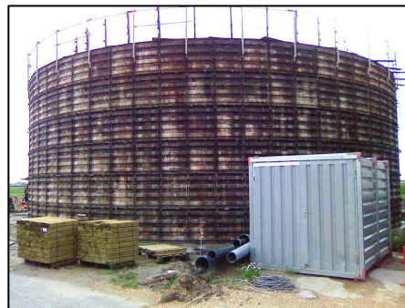
Figure 6-1 The construction of a manure tank at Nij Bosma Zathe.
