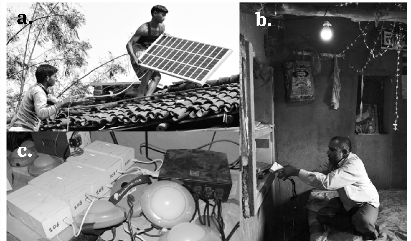
Figure 5 a, b, c, d. Photo: Abhigyan Singh. Energy Distribution Infrastructure. (a) Solar Panel. (b) Energy Router, Power banks, and Solar Lanterns. (c) LED Bulb and Power bank. Each solar item was imprinted with a unique numeric code to facilitate tracking of energy exchanges.
