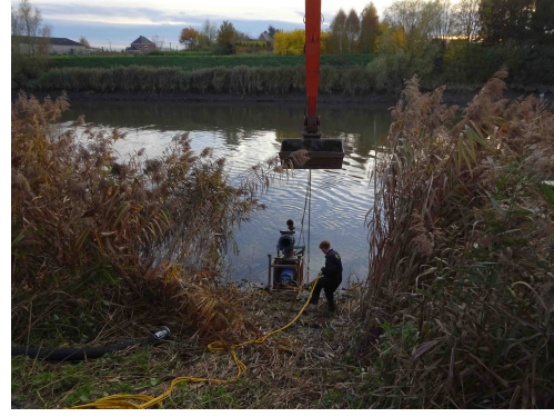
(B) Pump placed deep into the river water during low tide
