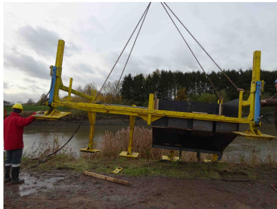
(C) Reservoir is supported by a steel frame
